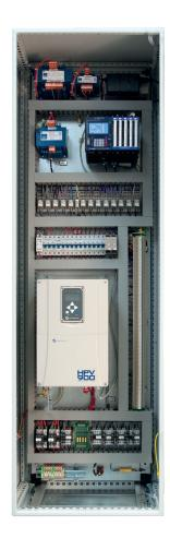
An easy-to-install AC drive, it provides accurate acceleration and deceleration, resulting in smooth ride quality. Magnetek's proven technical expertise and customer service are just two of the reasons why Lester Controls supply the HPV 900 S2. For geared installations we recommend the HPV 900 S2 every time.
